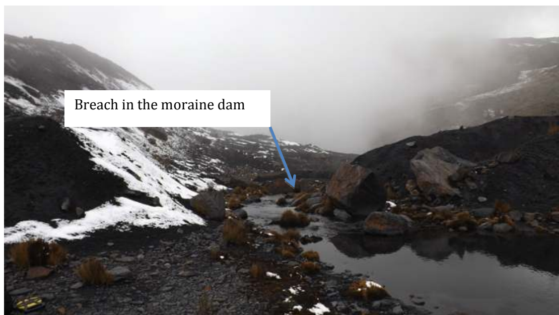
Figure 8 Breach in the moraine dam
