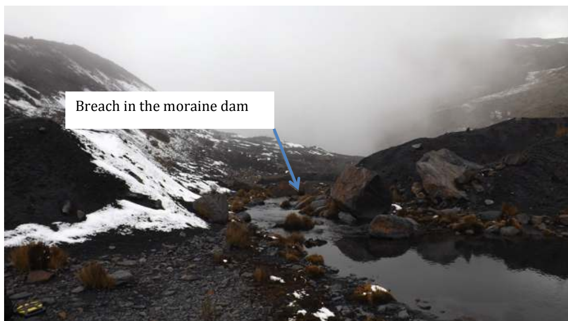
Figure 8 Breach in the moraine dam
